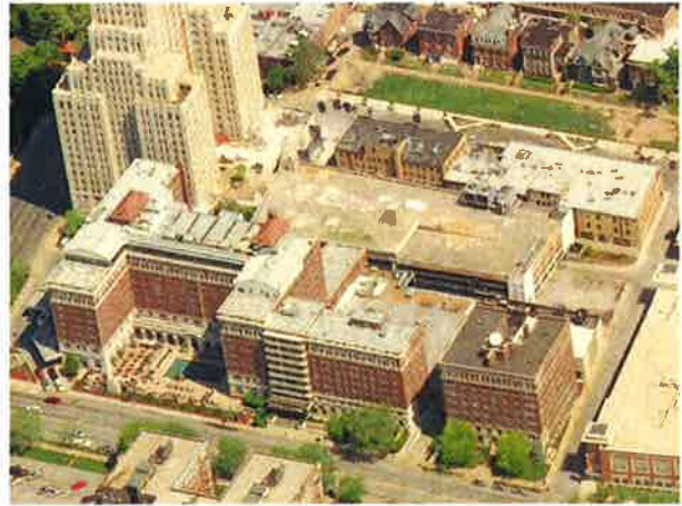
200 block of Forest Park Ave. Freestanding parking garage screen by buildings
