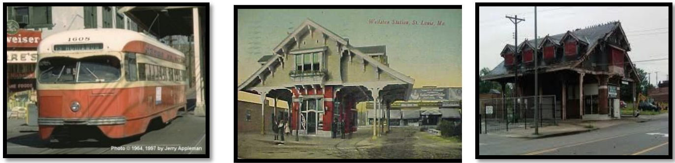
Wellston Loop Trolley; Wellston Loop Trolley Shelter in past years; Wellston Loop Trolley Shelter in current condition (Tate, 2012).
