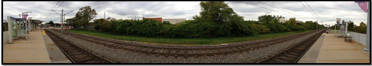
Wellston MetroLink Station, West Side of Tracks
