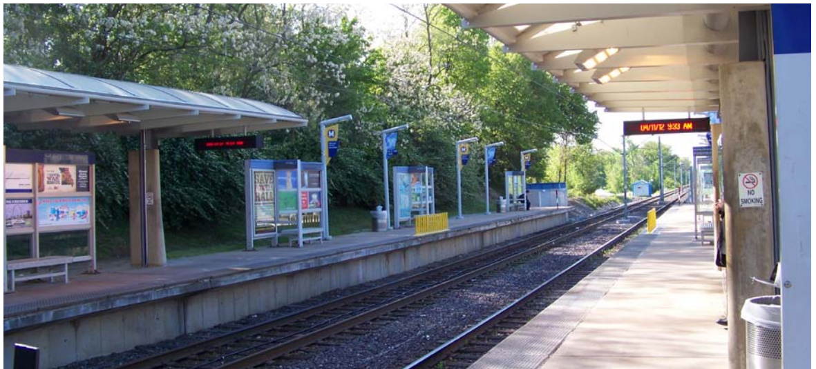
UMSL South MetroLink Station
