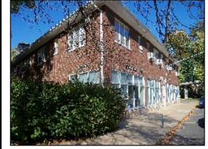
C: South of Pershing Ave.: Most of this neighborhood is developed with single-family homes, but some of the buildings adjacent to the MetroLink rail line are 2-story apartments and WUJSTL academic facilities.
