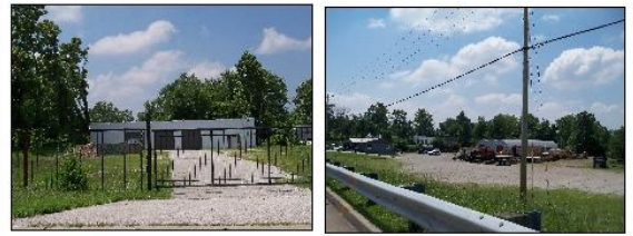
G - St. Charles Rock Road, east of MetroLink rail line: This mostly industrial block contains two industrial uses with small footprints on large lots, and one large vacant lot.
