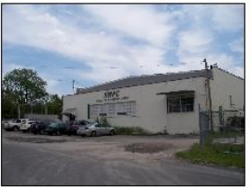
B- N. Market Street, west of MetroLink rail line: This block is occupied by three large, 1-story industrial businesses, most with surface parking and open storage.
