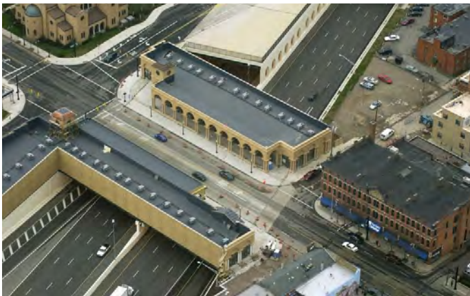
Short North, a new commercial development centered on High Street in Columbus, Ohio, effectively caps a major interstate, creates a retail and arts destination, and provides an inviting pedestrian experience for shoppers and students from The Ohio State University.
