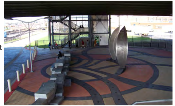
Plaza under Grand Avenue bridge, at station level
