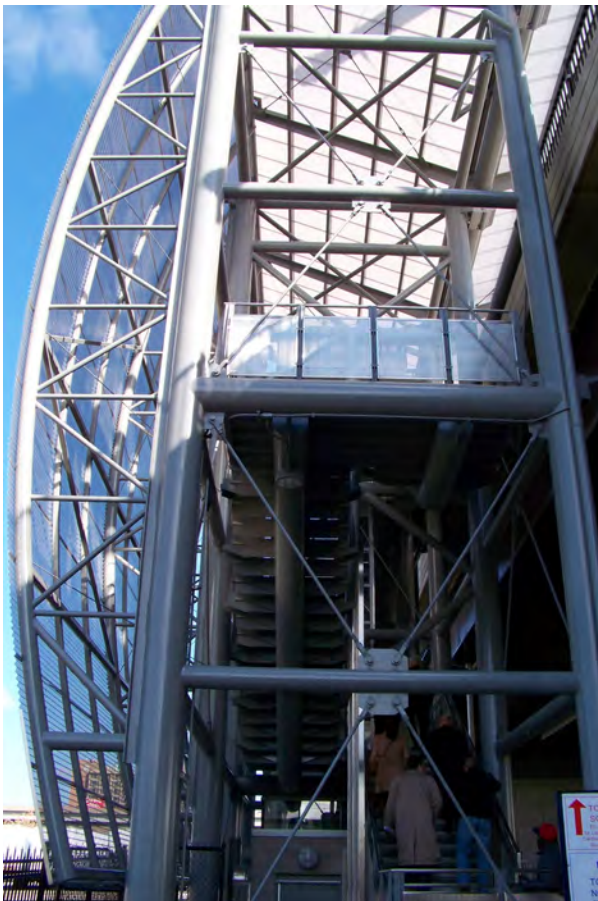
Stairwell connecting MetroLink station to bus platform on bridge above
