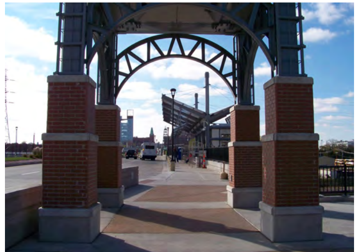
Archway welcoming pedestrians to Grand bus station platform
