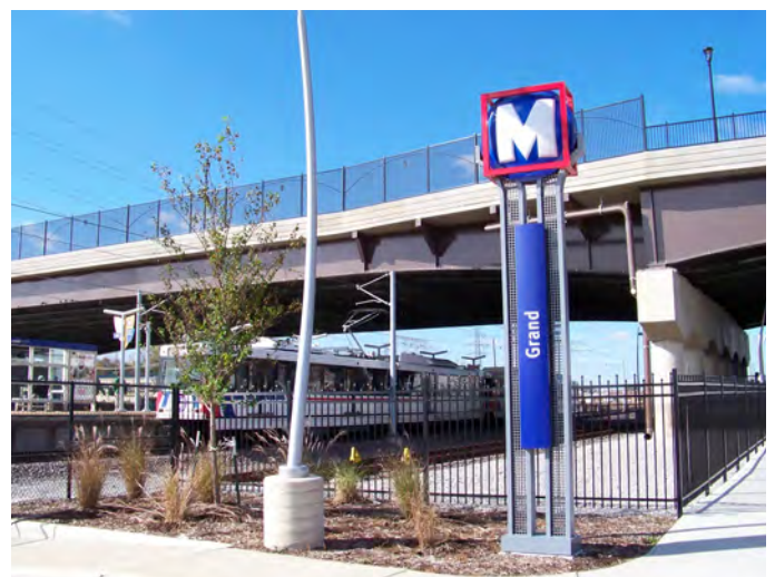
View of the station platform under Grand Avenue
