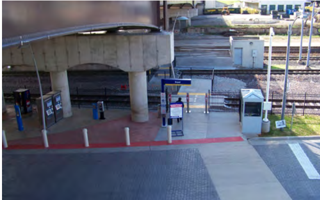
Station entrance, showing improvements to Scott Avenue
