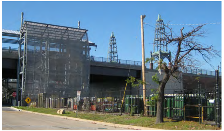
Stair access from station to Grand with Airgas adjacent
