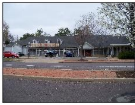
A - 500 DeBaliviere: 2 large community facilities, a 1-story retail strip, and three 2-story offices.
