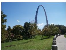
C - East of Memorial Drive, south of Washington Ave.: The entire southern portion of the station area covers the Jefferson National Expansion Memorial and Gateway Arch.
