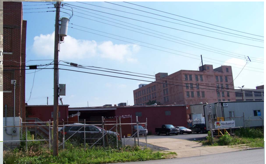
Site 2, View from Duncan
