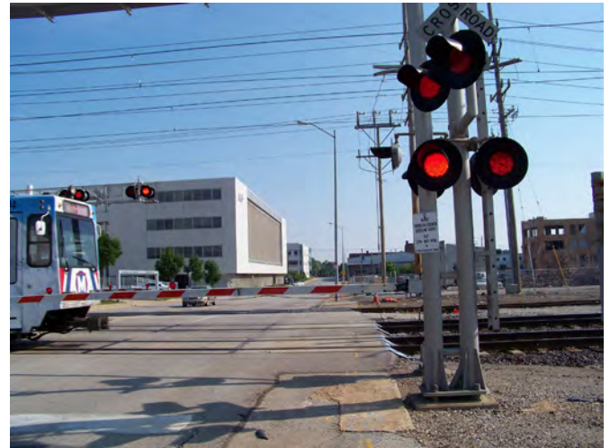
Intersection of MetroLink & Boyle, View to the North
