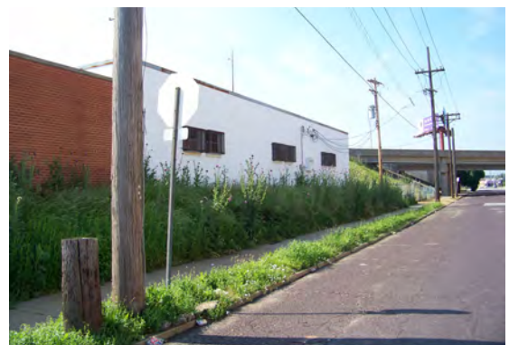
Southeast Corner of Sarah & Clayton Avenues
